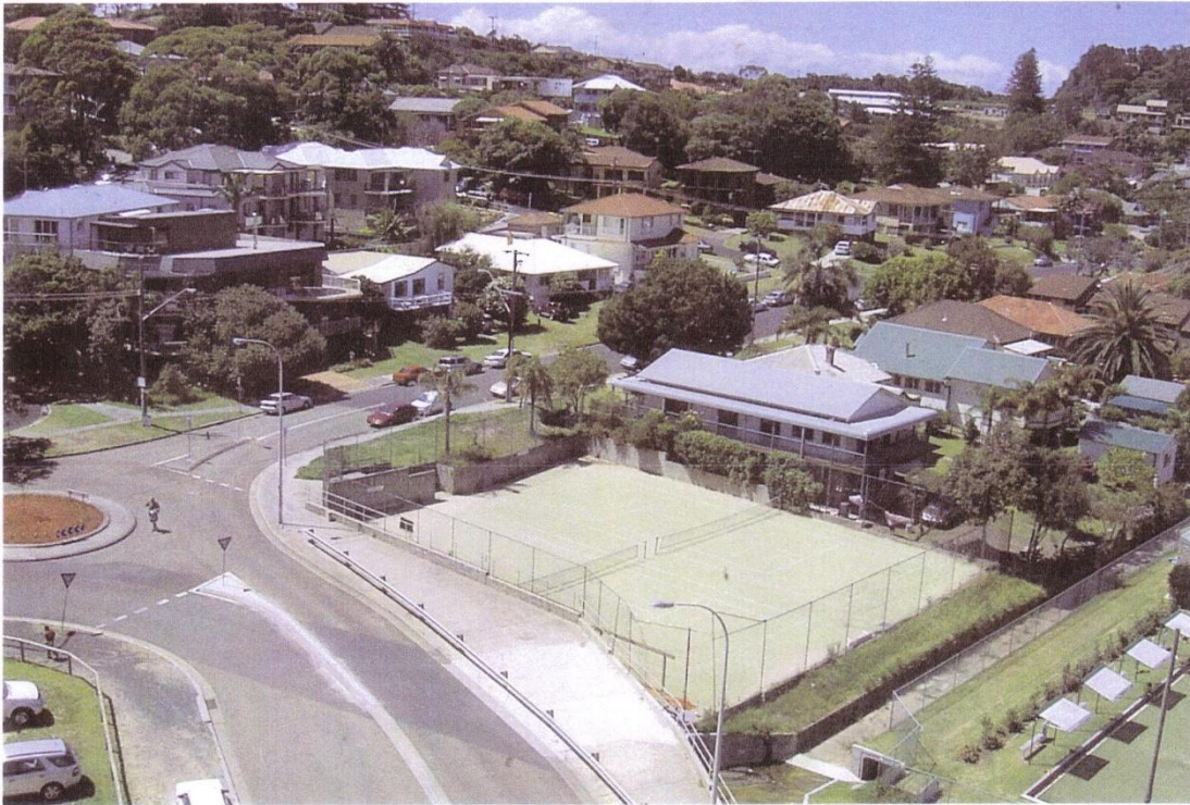
Photo 1: Subject land viewed from Crown Plaza Hotel
