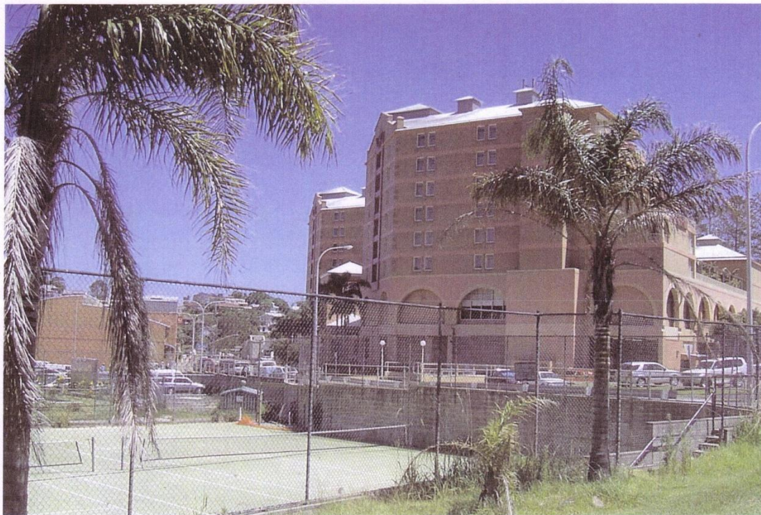
Photo 3: Subject land viewed from Ash Street looking toward Pine Tree Lane"
